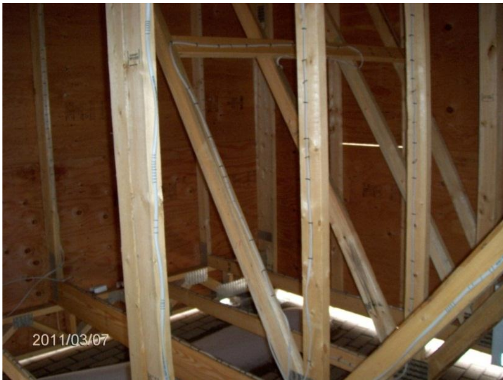
Figure 19 - NM cables installed on wood studs
